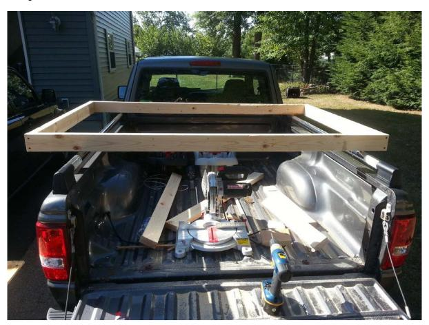
Once the frame was assembled I cut the plywood down to size and mounted it to the frame. Once this was completed the weight of the table quickly went up but so did the strength. Also, it is always advisable to have a helping hand when building anything, especially when it comes to using power tools. As you can see my helper Jake is very proud of the work he did using a screw gun.
